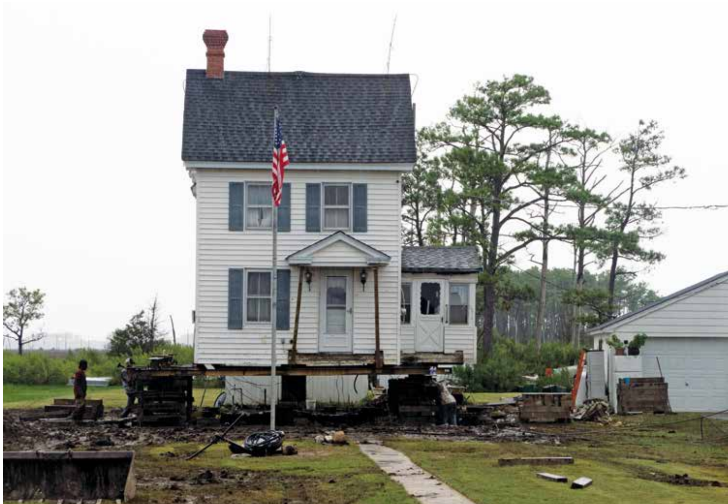
This property in Dorchester County, MD, flooded regularly during full-moon high tides and other tidal events. In 2017, it was raised 8 ft. David Harp/ChesapeakePhotos.Com.
