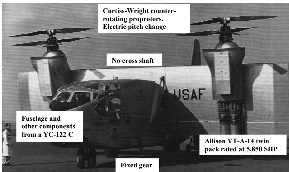
Fig. 2-81. The Hiller X-18 tiltwing 33,000-pound experimental aircraft first flew on November 24, 1959. It had so many propotor, engine, and other design problems that the U.S. Air Force cancelled the program on January 18, 1964.
