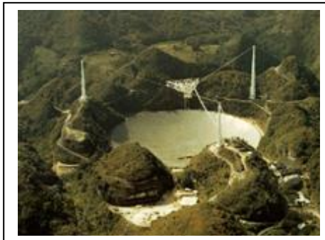
Figure 6: The Arecibo radio telescope. The spherical primary reflector is 1000 ft in diameter. A line feed for 400 MHz operation can be seen hanging below the platform and track. The tip of the line feed is at the paraxial focal point of the spherical primary.
