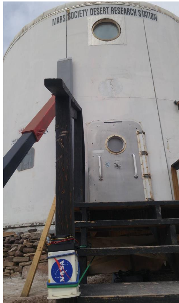
Figure 20: SFS' SMF location mounted outside of MDRS for Test #11 to measure passive dust collection over two hours.
