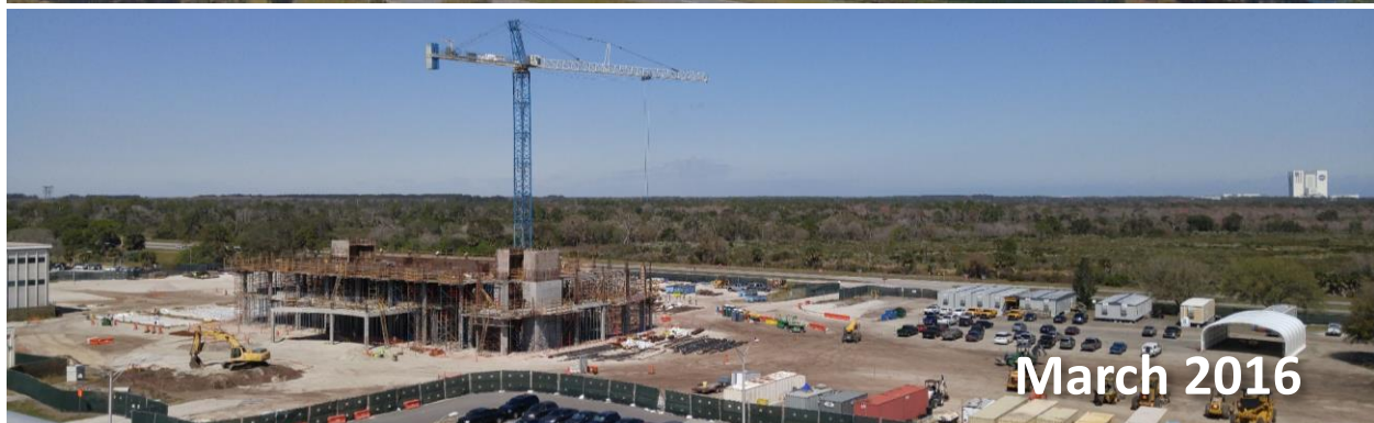
Central Campus Headquarters Phase I Construction
