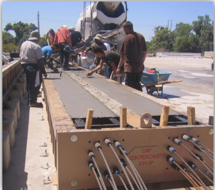
Precast Test Piles Production - Deland Precast Plant
