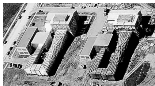
Building N-215 with 7- by 10-Foot Subsonic Wind Tunnels (circa 1940).
