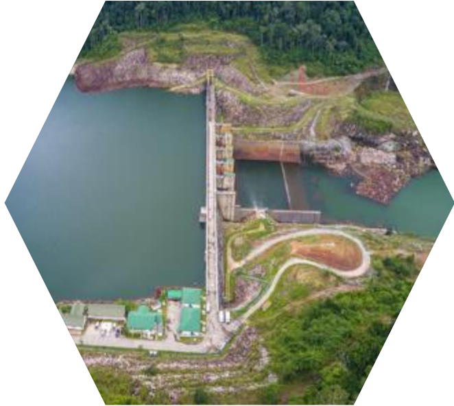
Dam on Nam Theun river in Laos
