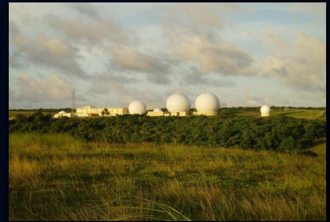
Guam Remote Ground Terminal
