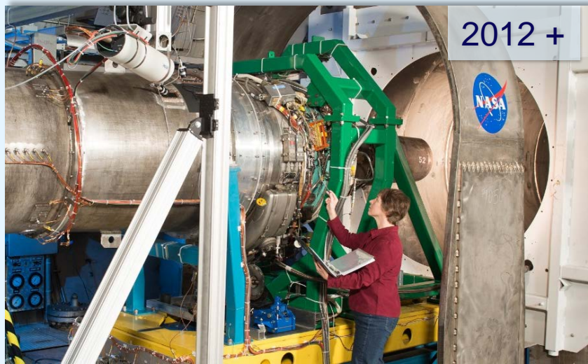
Propulsion Systems Lab, PSL
