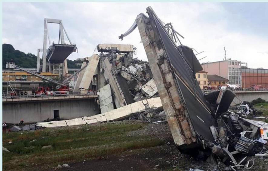
Genoa bridge collapse
