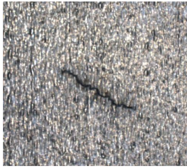
Laser cut crack
