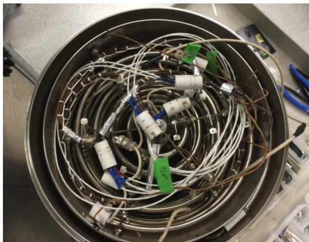
Figure 6: The CRCSb heating coils inside the stage 1 and stage 2 cylinders.
