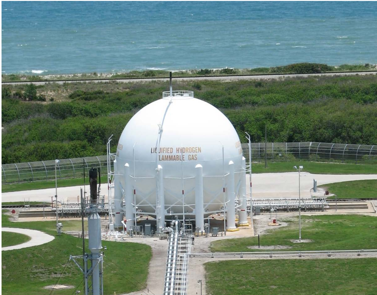
Figure 1. Liquid hydrogen storage sphere at NASA's Kennedy Space Center
