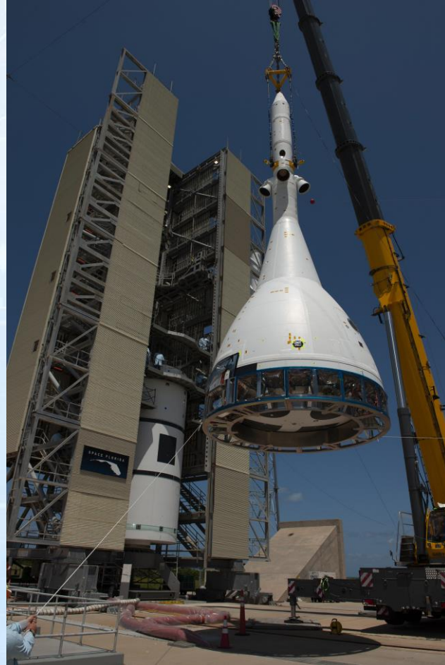
Assembly at KSC
