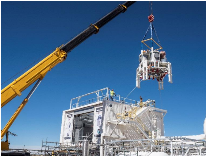
Figure 2: PQM Being Installed at WSTF TS-301
