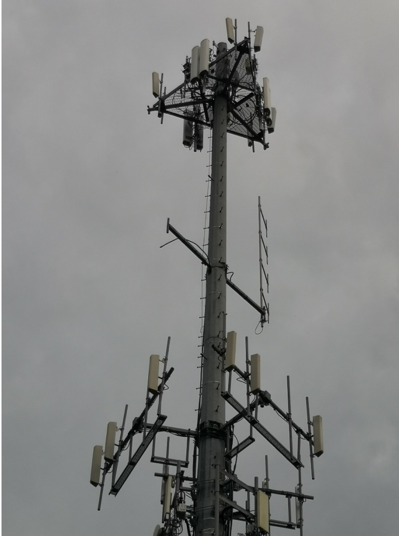
A Verizon Base Station with Sector Antennas
