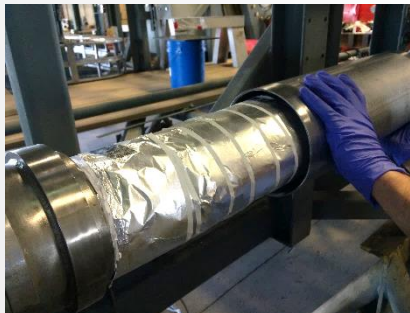
MLI wrapping in the shop
