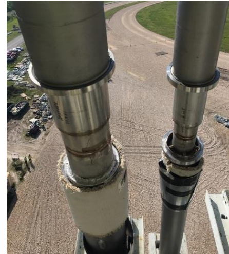
Before close-out with cans and aerogel in the field
