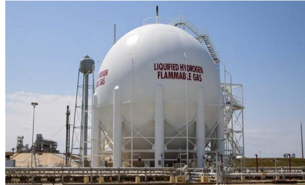
2) Large spherical tank: moderate vacuum ( \sim 10\mu )
