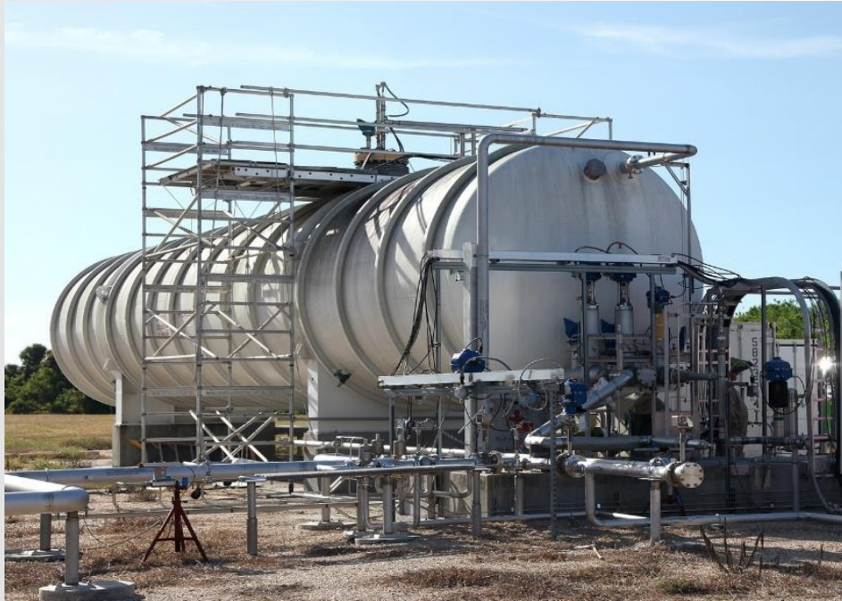
1) Medium cylindrical tank: high vacuum ( <0.1\mu )
