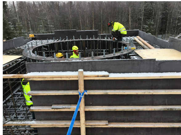
Fig. 1 Foundation construction and installation of the anchor ring.
