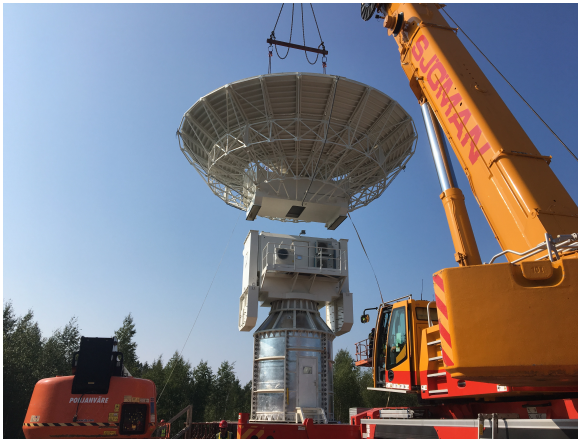
Fig. 3 Assembly of the radio telescope.
