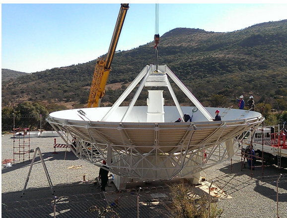
Fig. 3 Assembly of the main reflector.
