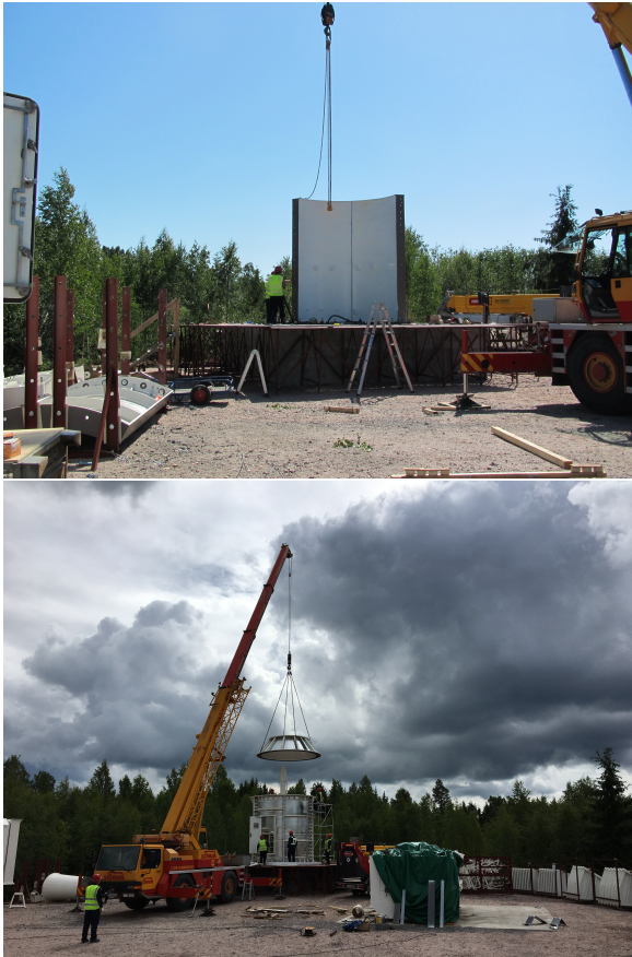
Fig. 2 Assembly of the steel pedestal.
