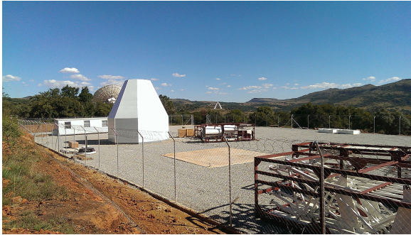
Fig. 2 The finished concrete base.
