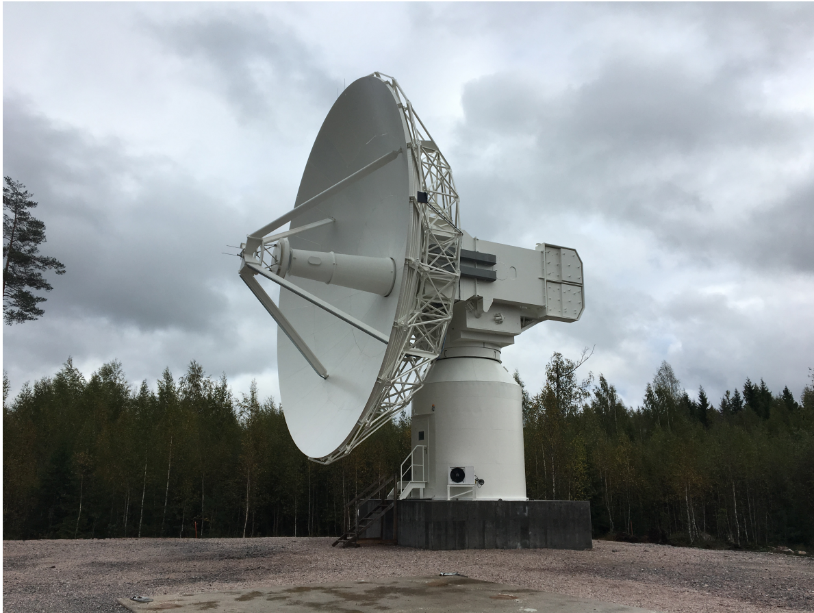
Fig. 4 The VGOS radio telescope installed at Metsähovi.
