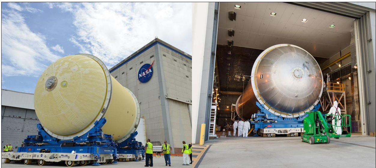
Fig. 6. EM-1 LOX tank moves after thermal protection foam application, left. The LH 2 tank moves into a manufacturing cell for priming and thermal protection foam, right.
