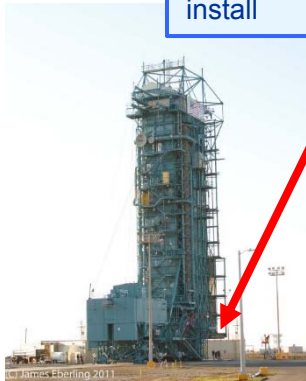
Mobile Service Tower (MST) in place (around vehicle) for Integration and Fairing install
