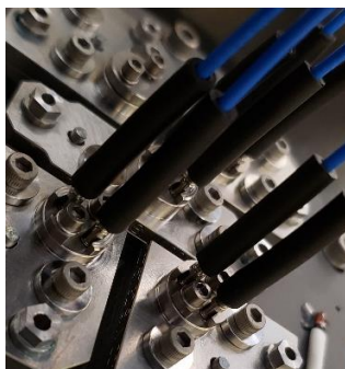
Figure 12a: Fibers installed to RTA
