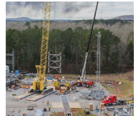
Construction of 2 nd SLS test Stand
