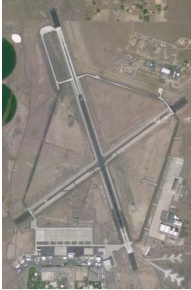
Figure 9. Grant County International Airport satellite view.
