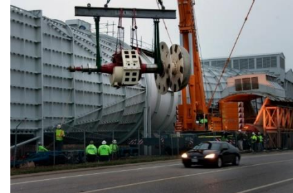
Removal of main drive
