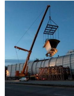
Removal of part of the nacelle and tunnel structure
