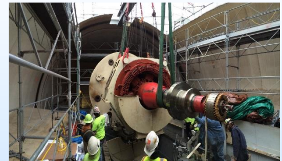
Removal of drive motor
