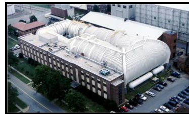
LaRC Transonic Dynamics Tunnel Aeroelasticity & Flutter
