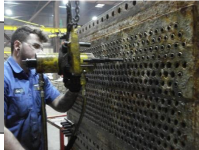
Heat Exchanger Module Prep
