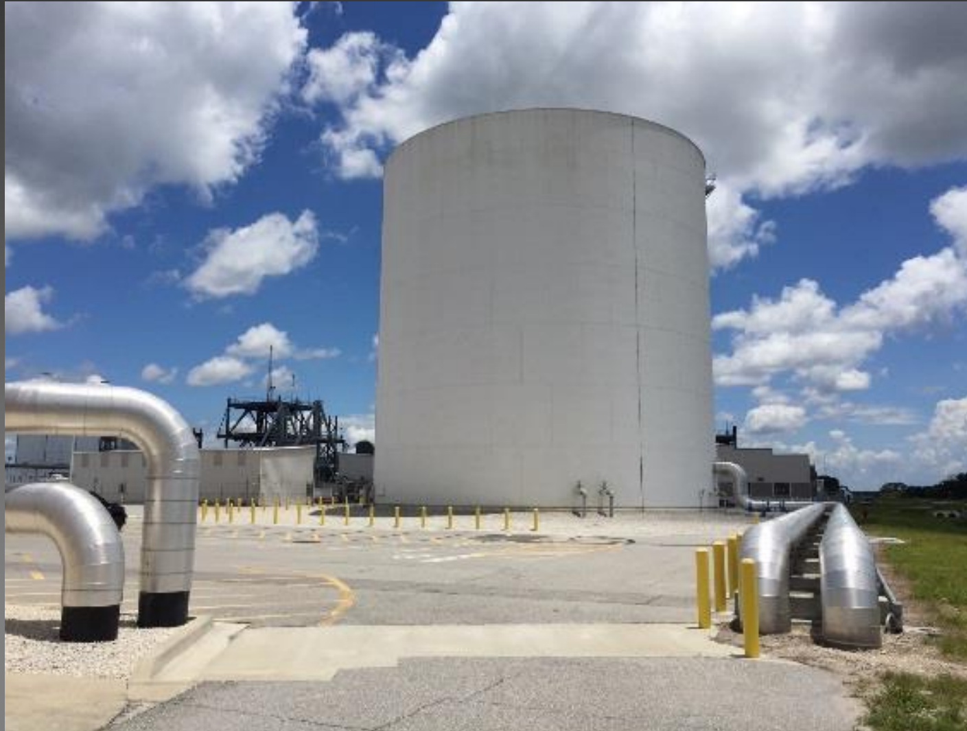
Fig 1. KSC Industrial Area Water Tank
