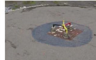
Completed Landing Pad
