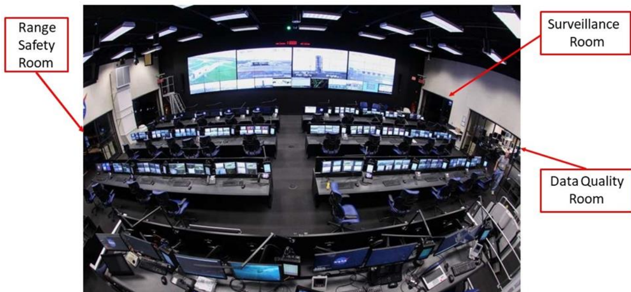
Figure 6.2-1. WFF RCC Mission Control Room
