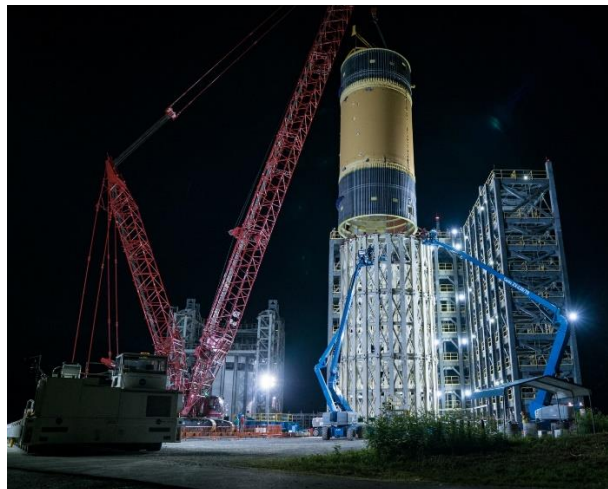
Fig. 8. LOX structural test article during installation
