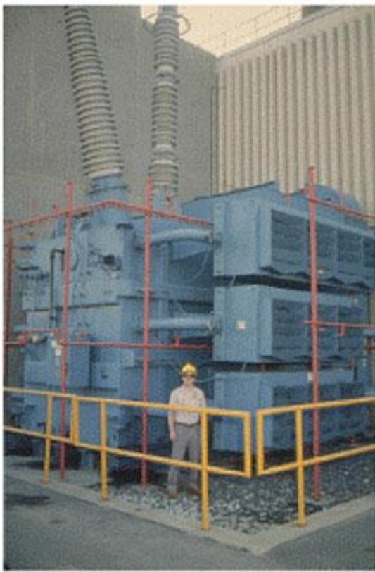
Permanent damage to the Salem New Jersey Nuclear Plant GSU Transformer caused by the March 13, 1989 geomagnetic storm. Photos: PSE&G
