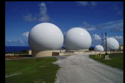
Guam Remote Ground Terminal
