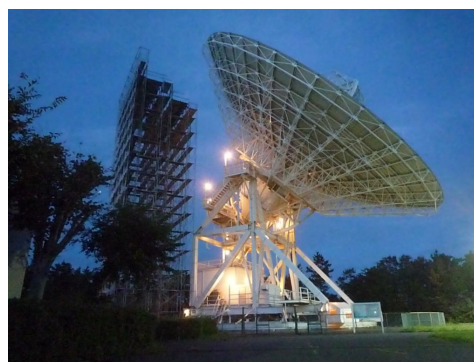
Fig. 6 The Kashima 34-m antenna in holographic observing after reflector adjustment. We carried out the reflector adjustment during day time and the holography observing in the evening. We repeated this procedure for a week. For safety, we watched the antenna during the holography observing for about 1.5 hours to avoid an accidental smash with the scaffolding.
