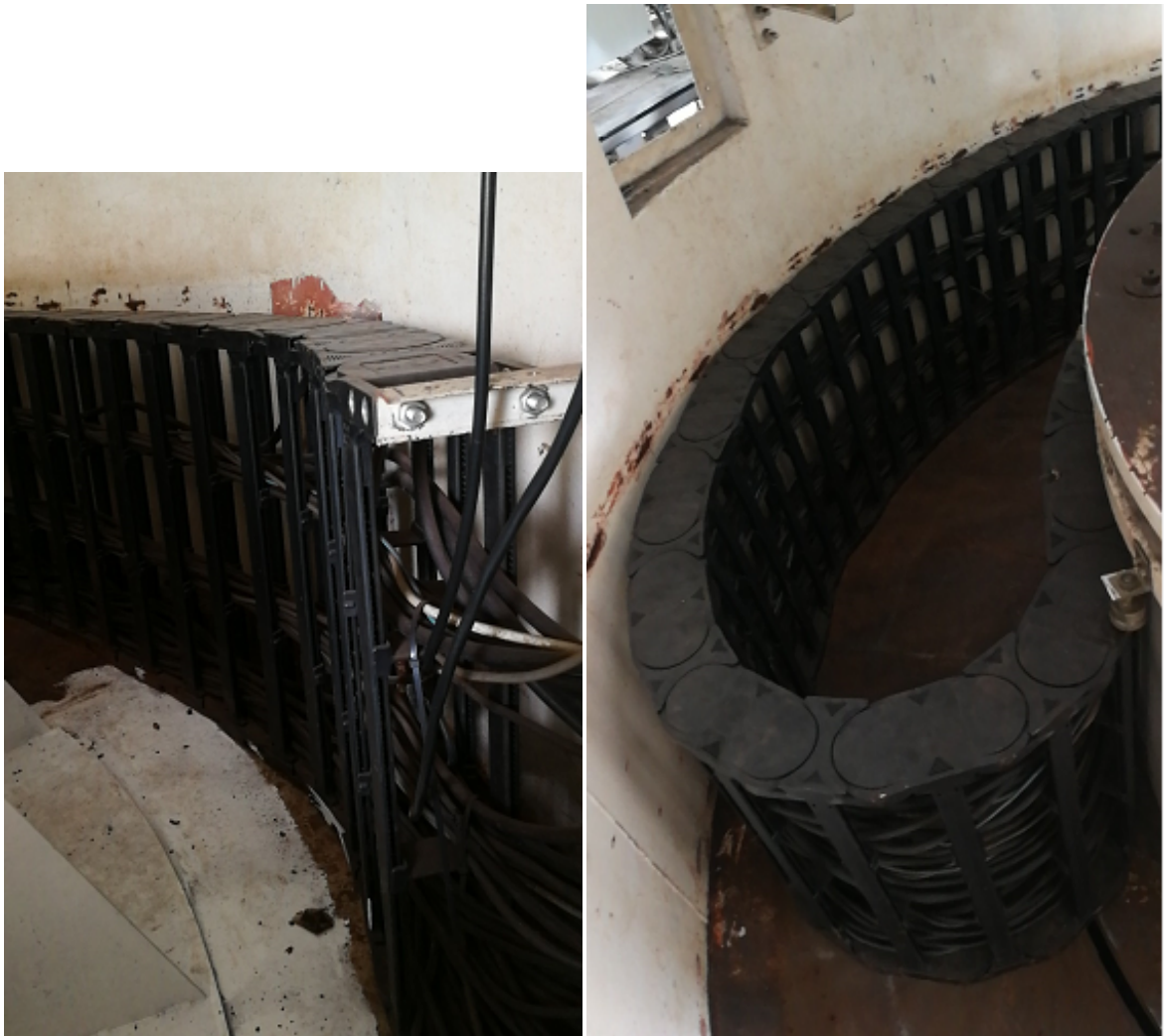
Fig. 2 The antenna maintenance of the SHESHAN 25-m telescope.
