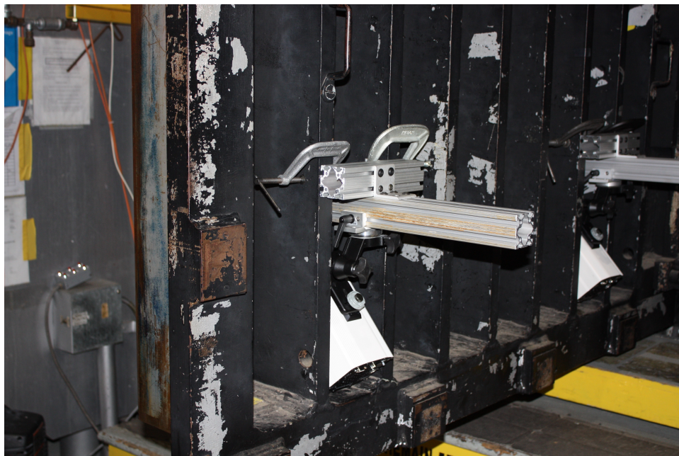
Fig. 10 Mounting of PSP cameras on the tunnel door webbing.
