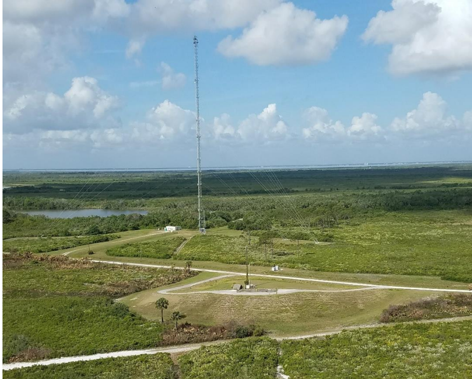
Figure 70. Primary array site and tower J6-0490A. Small hill in foreground was mini SODAR location and GPSsonde launch point.
