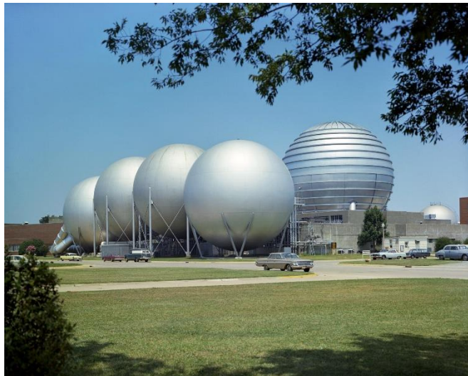
Figure 3. Langley's Gas Dynamics Laboratory with multiple hypersonics test facilities.
