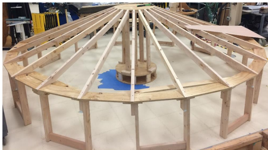
Mock-up Heat Shield Framing
