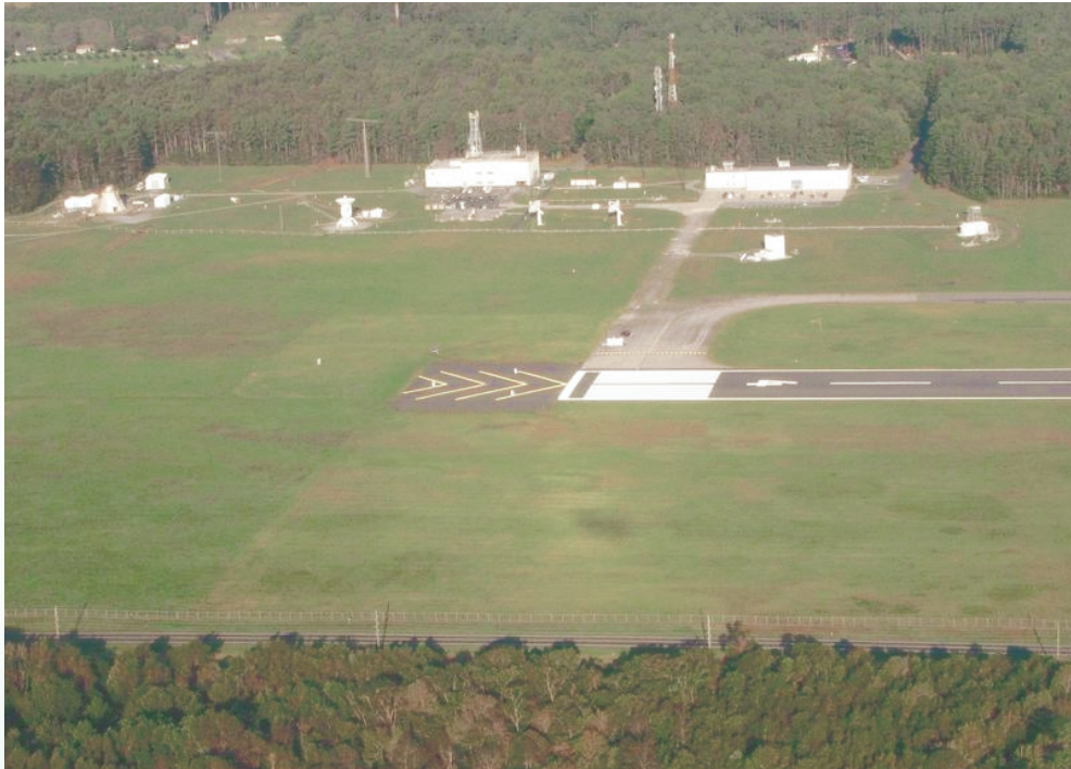
WFF Runway 4 Threshold Area
