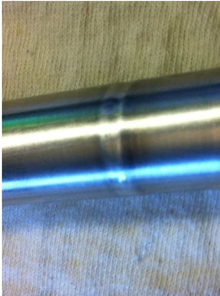
Lack of Fusion
