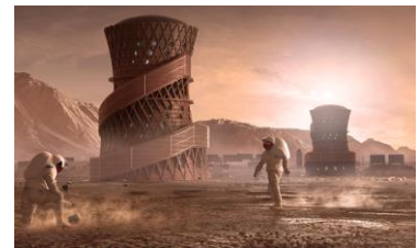
Figure 1. Team SEArch+/Apis Cor won first place in the Phase 3: Level 4 software modeling stage of NASA’s 3D-Printed Habitat Challenge. The unique shape of their habitat allows for continuous reinforcement of the structure. Light enters through trough-shaped ports on the sides and top. (Image:Team SEArch+/Apis Cor)
