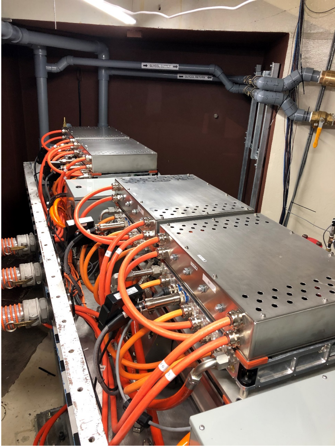
Fig. 3: Dynamometer Table without Shroud Lid Installed
