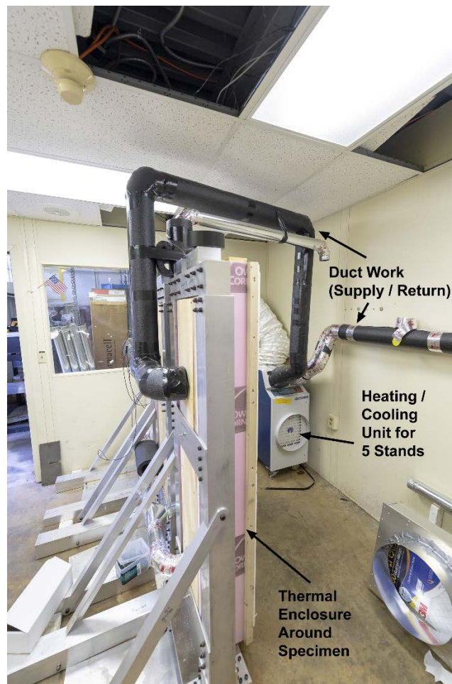
Figure 8. Thermal enclosure with ductwork.
