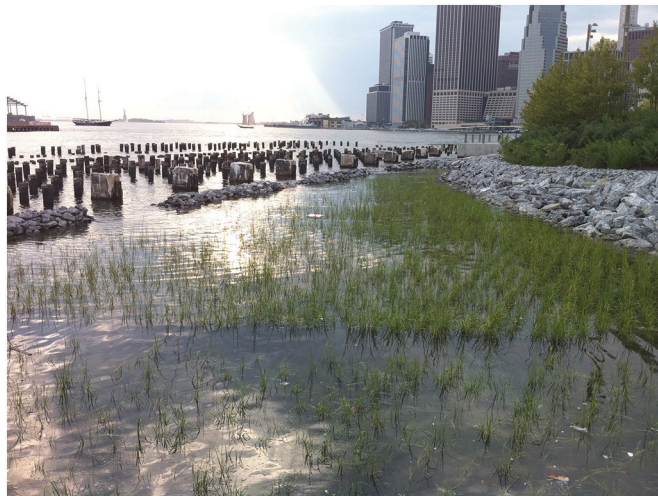
Fig. 8. Soft edge “living shoreline”, Brooklyn Bridge Park, New York City. (Source: New York City Department of City Planning, 2013).
