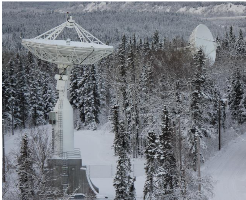
Figure 7-3. AS3 Antenna and Foundation (foreground) Existing AS1 (background)
