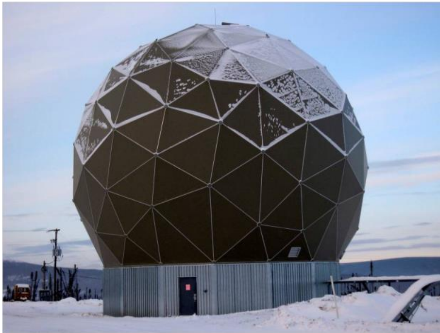
Figure 6-4. USAK05 Antenna Radome
