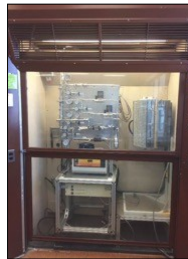
Gas flow panel and furnace in fume hood
