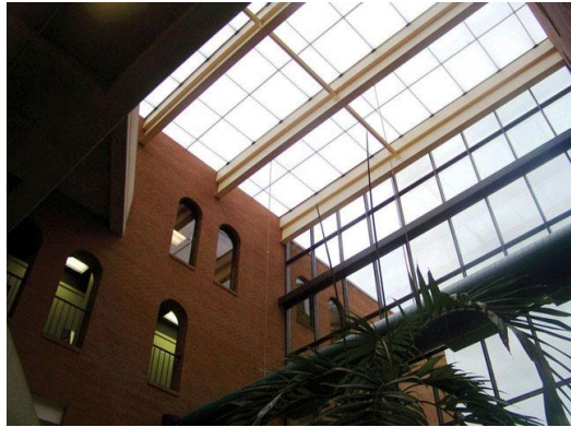
Cabot Lumira Aerogel in skylights Grand Rapids, Mi
