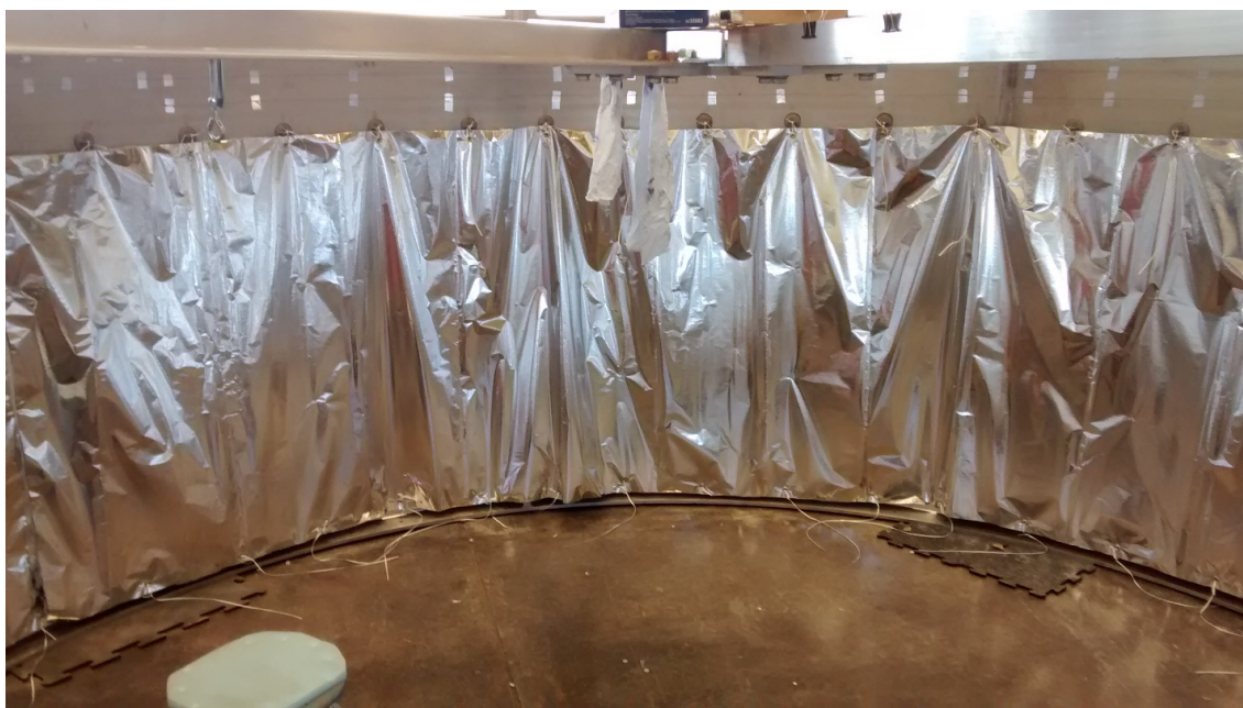
Figure J.10.—Multilayer insulation installed on the aft skirt.
