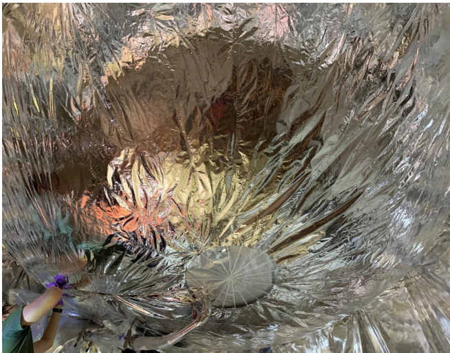
Figure J.15.—Installation of the third subblanket onto the aft dome.
