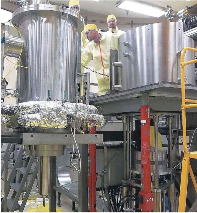
Fig. 3. The vacuum chamber (left) containing the core (inside lower left) and PCS (inside upper left) is lifted to be installed on COMET (right), which holds the large SS304 shield (upper right) and the lower shielding on the platen (lower right).
