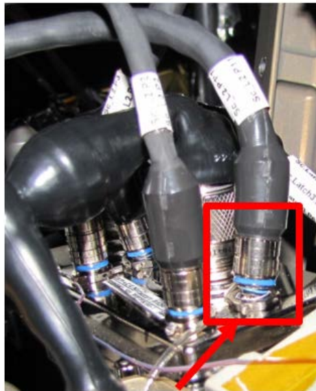
Figure 10: Harness Connector Sheared during Deployment
