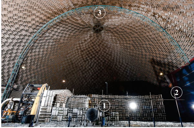
Fig. 2 DART ①, sideline ② and overhead ③ arrays
