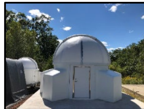
Dome Construction at Millstone Hill
