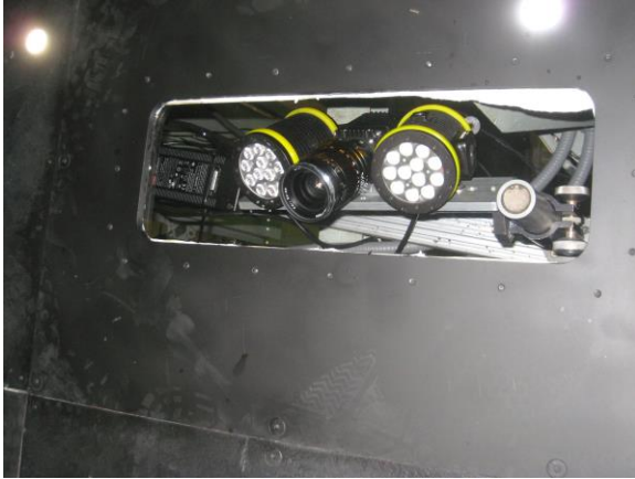
Fig. 4 Camera and lamps installed at one window in turntable.
